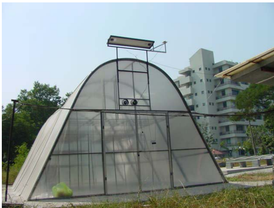
Figure 6.15. The greenhouse solar dryer. ( Janjai et al. 2007 )
